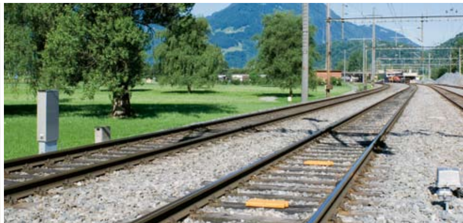
Transmission point with Trainguard Eurobalises S21
